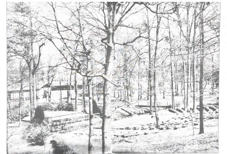
TIMROD PARK AMPHITHEATER –View in city park showing the stage and seats of the outdoor theater in 1938.
