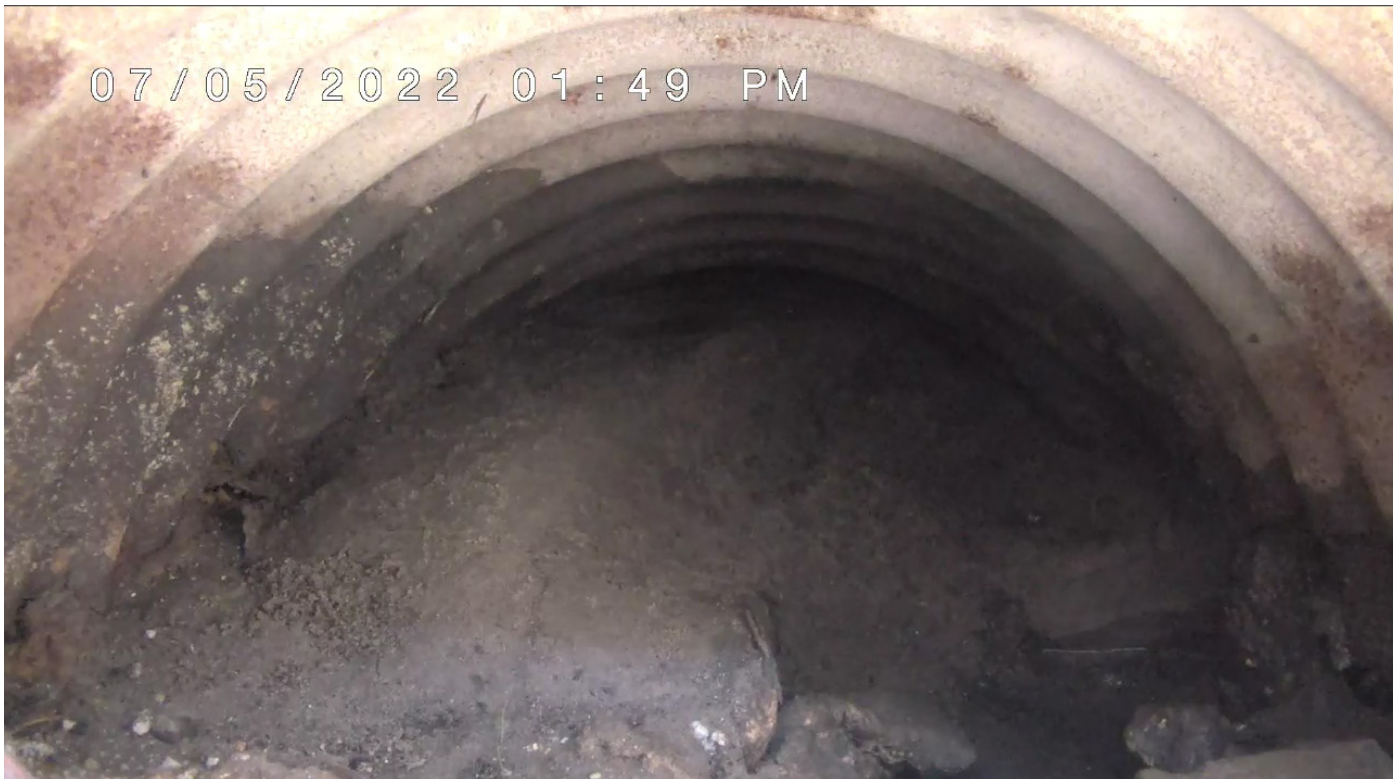
Figure 12: Structure 17 line blockage
