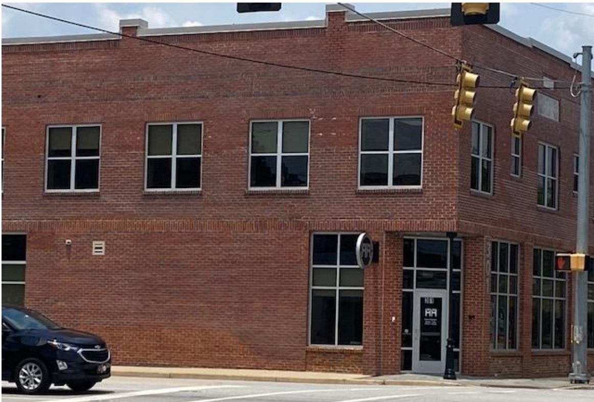
Windows on the Streater Building at 301 North Dargan Street.
