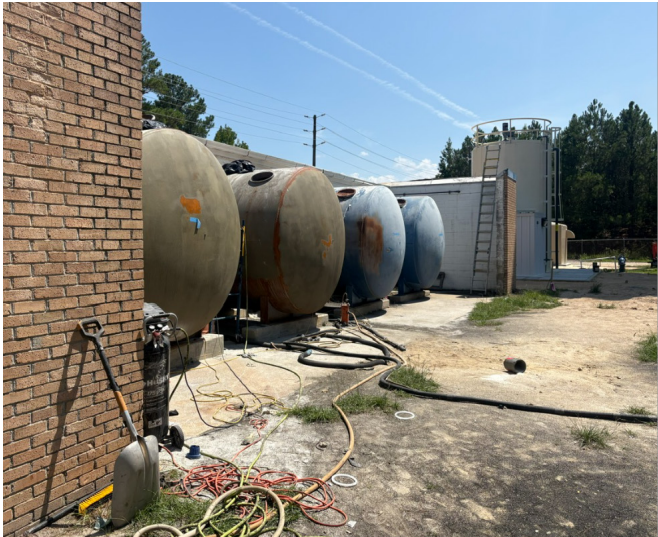
1 SCIIP GE Groundwater Treatment Plant Upgrades
