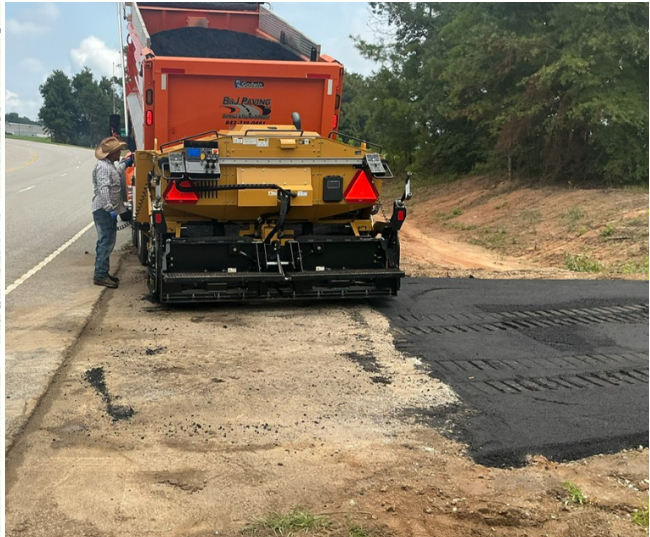
3 Freedom Blvd Waterline Extension
