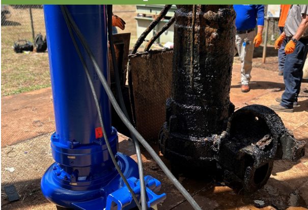
2 East Florence Lift Station Improvements
