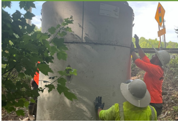
1 Jeffries Creek Sewer Manhole Raising
