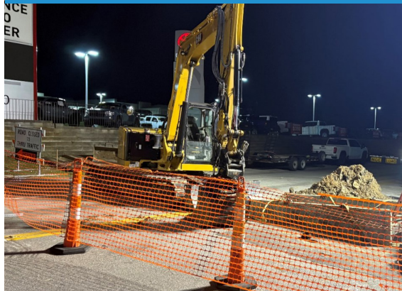
2 Holly Circle Waterline Relocation
