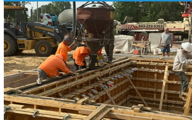
5 SCIP GE Ground Water Treatment Plant Upgrades
