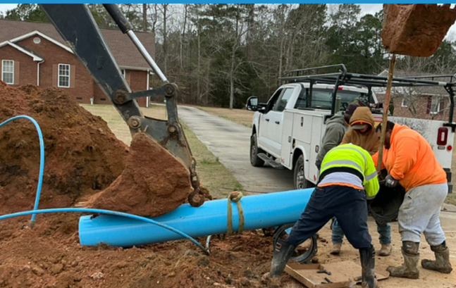
3 Paper Mill Road Utility Relocation
