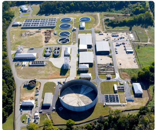
Aerial view of the City's regional wastewater management facility, located at 1000 Stockade Drive.
